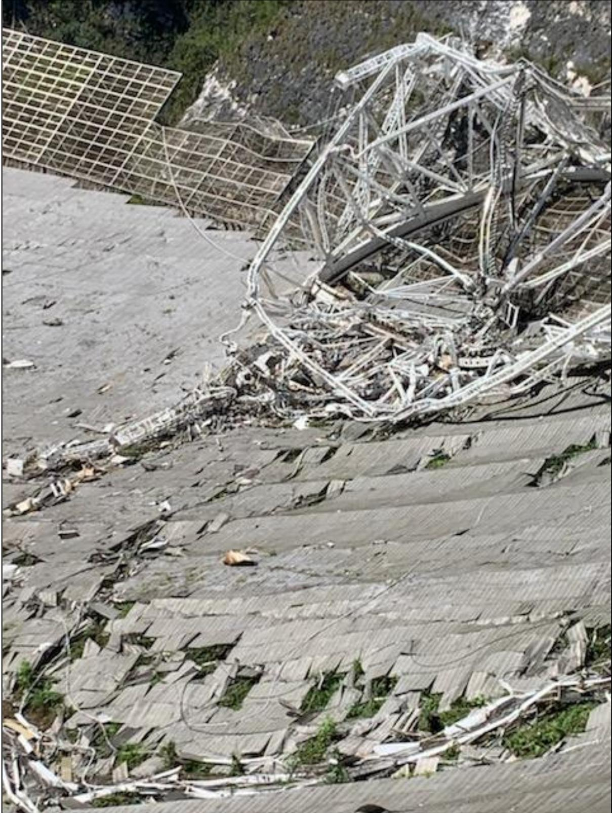
Twisted steel and damage sustained to the dish from the falling receiver
