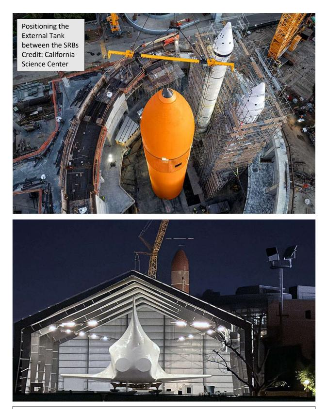
Space shuttle Endeavour, covered in shrink wrap, waits to be lifted and stacked while the crane moves the External Tank in the background. Photo: Matt Hartman/Shorealone Films
