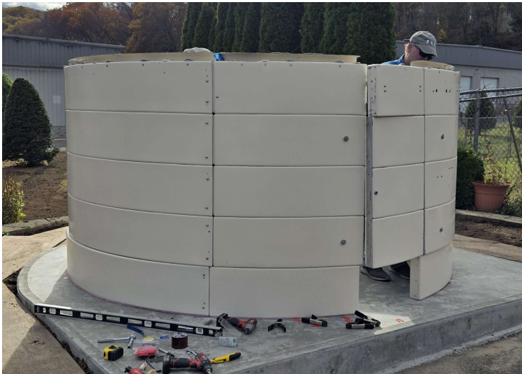
From top left: pier footing with electrical/communication conduits, first dome ring positioned on concrete pad, wall assembly, dome installation, and initial telescope placement
