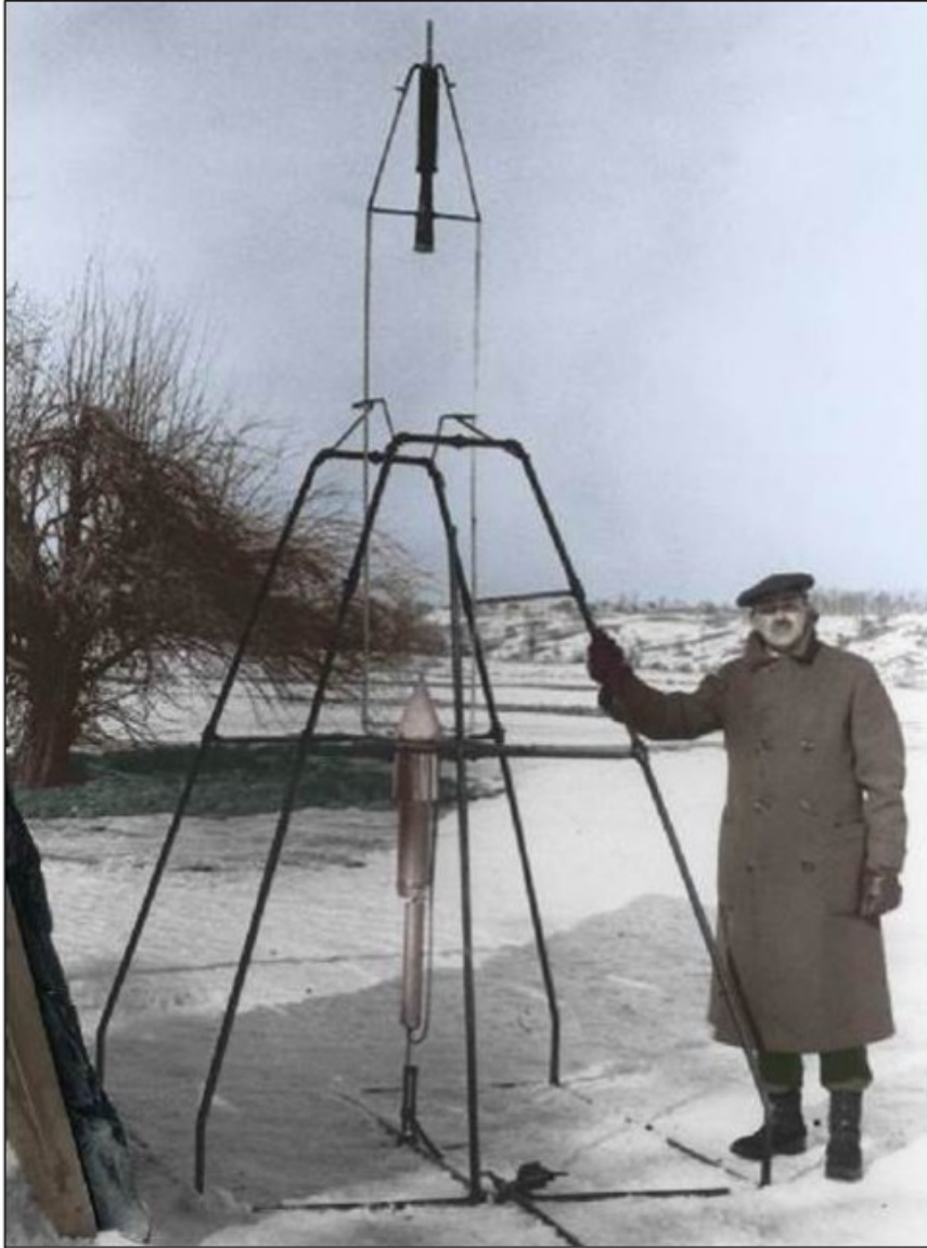
Dr. Goddard with his liquid oxygen-gasoline rocket "Nell" in its launching frame
