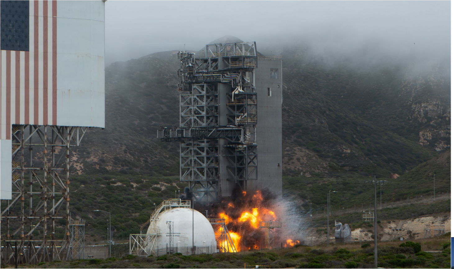
Explosive demolition of launch pad SLC-6 U.S. Space Force photo by Staff Sgt. Daekwon Stith
