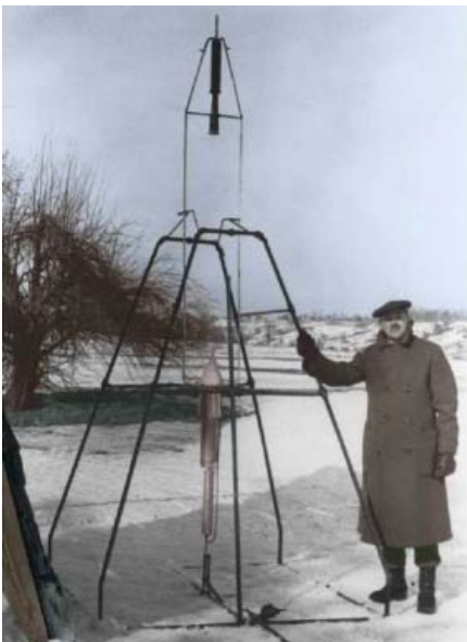
Dr. Goddard with his a liquid oxygen-gasoline rocket "Nell" in its launching frame (NASA photo).
