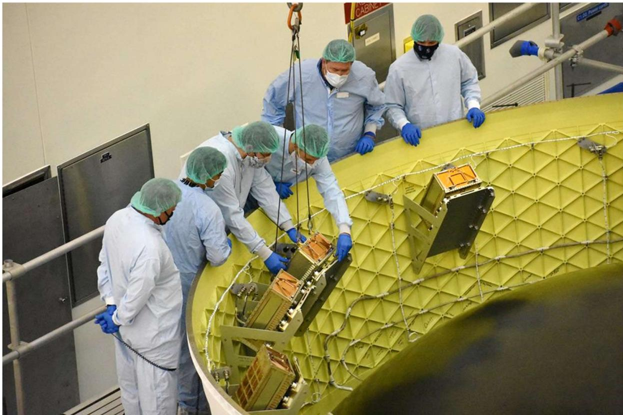
Technicians installing the last of 10 CubeSats in the Space Launch System (SLS) rocket’s Orion stage adapter for the Artemis 1 flight in November 2022.
