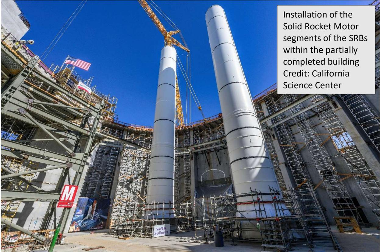
Installation of the Solid Rocket Motor segments of the SRBs within the partially completed building
